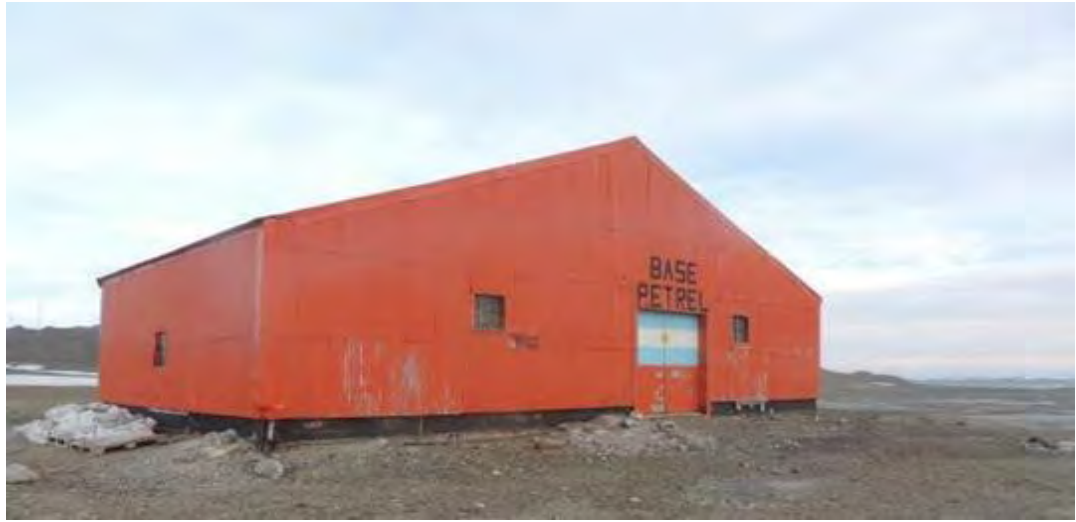
Figure 8: General view of Warehouse I
