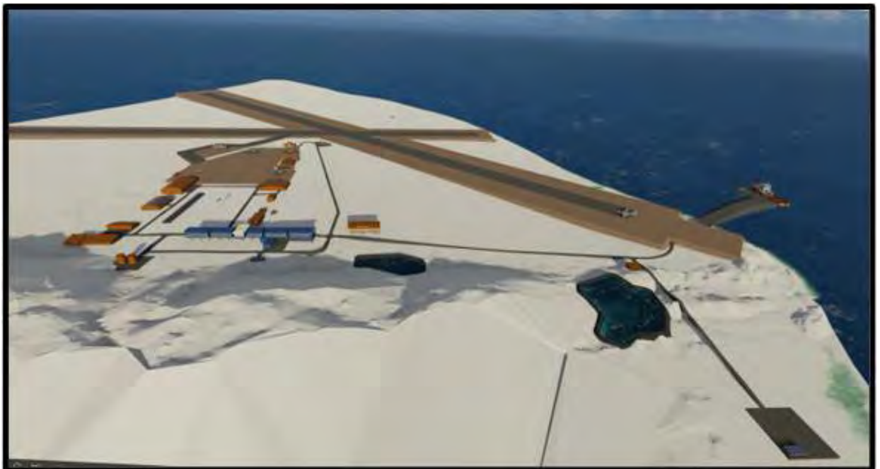
Figure 21: Original general design of the new Petrel Base.
