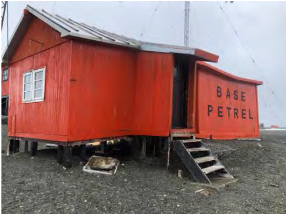
Figure 11: General view of the Power Plant (in disuse)
