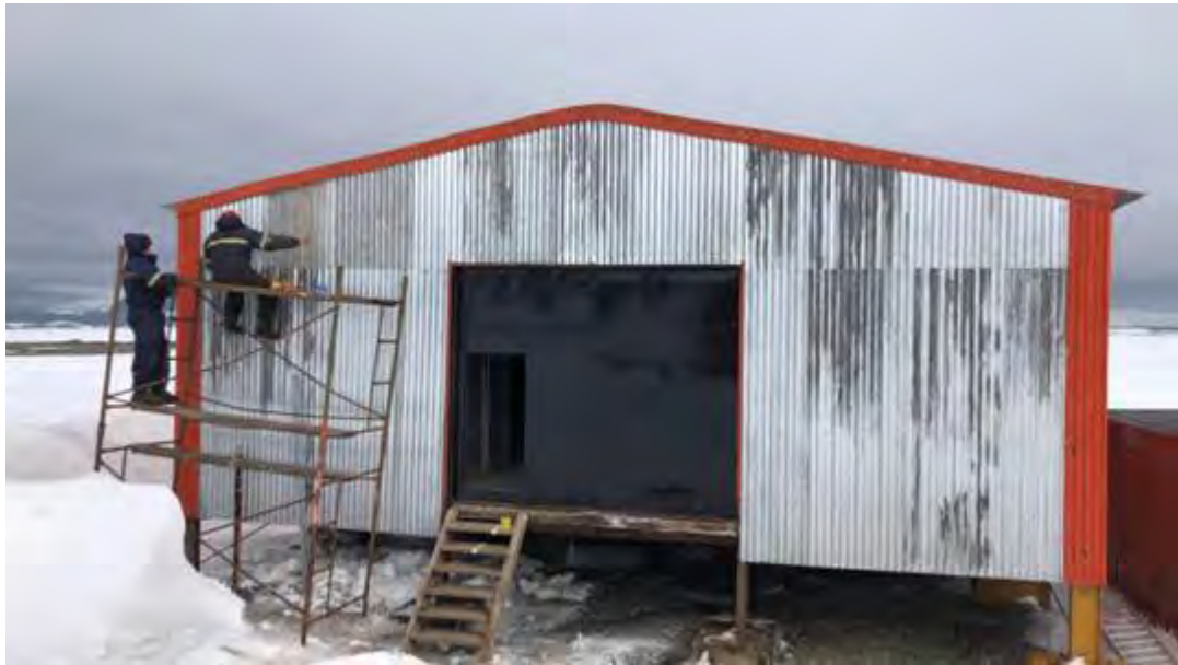
Figure 16: Maintenance tasks carried out in the 2022 Campaign in Warehouse II.
