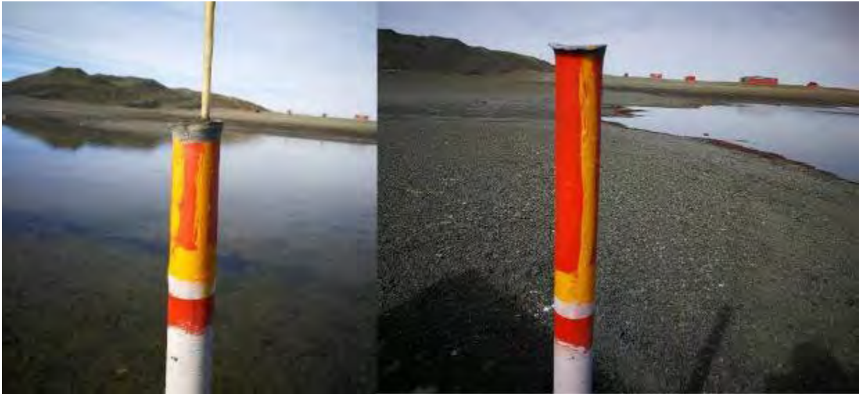
Figure 121: Marking with a yellow ring to measure upwards the fill height necessary for the project.
