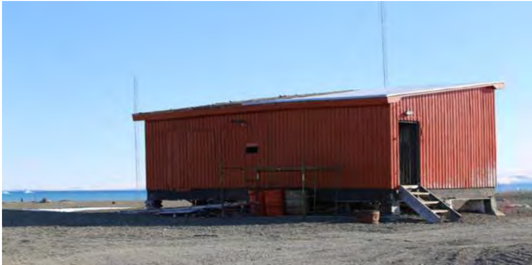
Figure 9: General view of the former power plant (emergency power plant).
