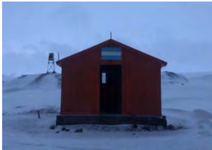
Figure 12: general view of the Port Depot.
