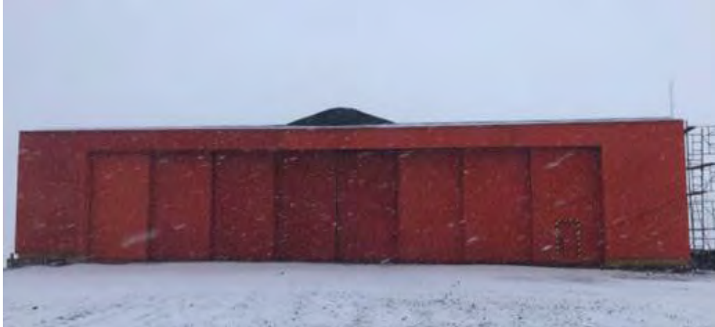
Figure 15: Current state of the Hangar after the maintenance and conditioning tasks carried out in the 2022 campaign.
