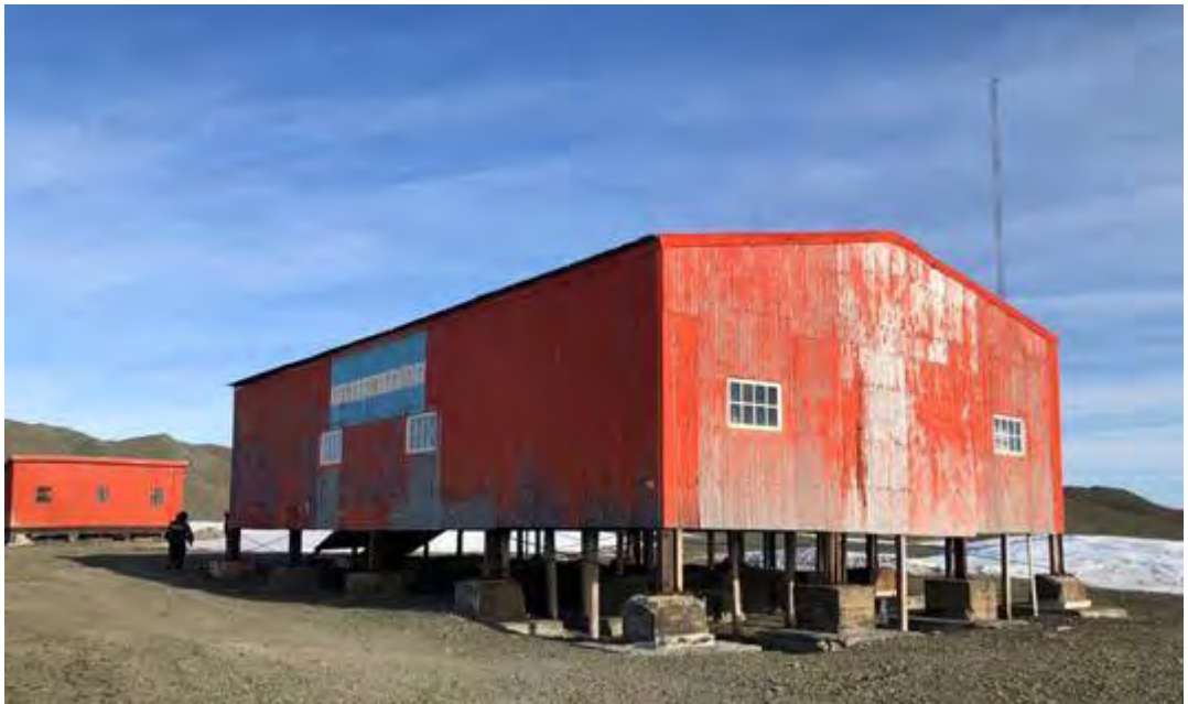
Figure 8: General view of Warehouse II
