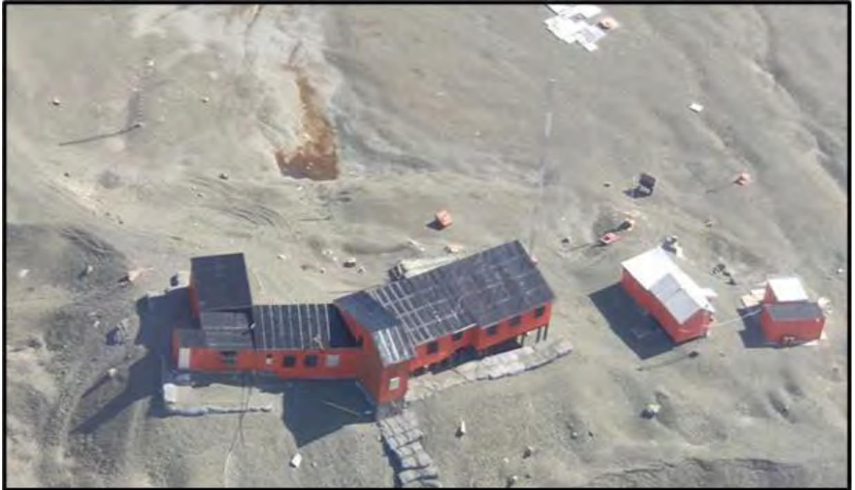
Figure 6: General view of the Main House.
