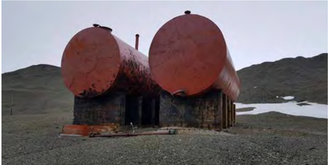
Figure 17: Current status of the tanks at Petrel Base.
