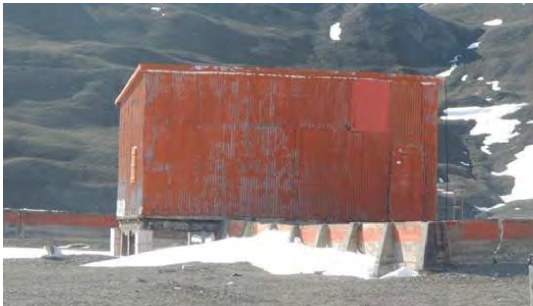
Figure 10: General view of the Cold Room.
