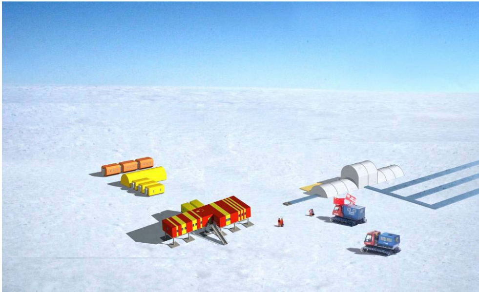
Fig. 16 Bird's-eye view of the Station construction
