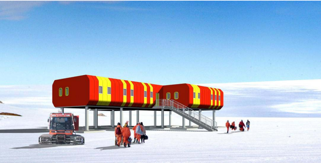
Fig. 15 Main Building of the station
